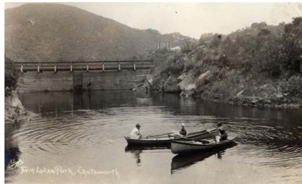
Twin Lake residents boating on Raymond Lake. The Dam shown on the left is still in place and serves as an access bridge to homes north of Devil Canyon. The dam gate was opened in April of 1948 after much discussion of required maintenance and with some hesitation, not knowing if it would refill with the next rain season.
